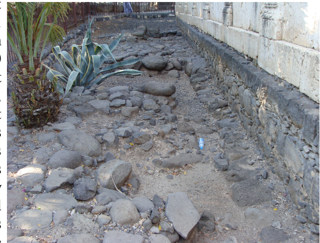
Foundation stones of the synagogue in Capernaum that the centurion helped build
